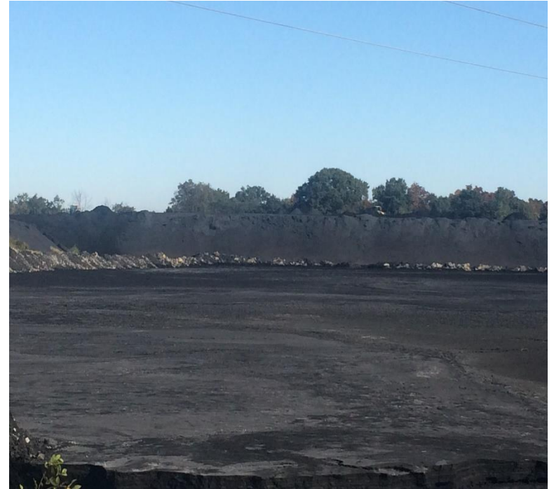
Riceland Temporary Storage. Stuttgart, AR
